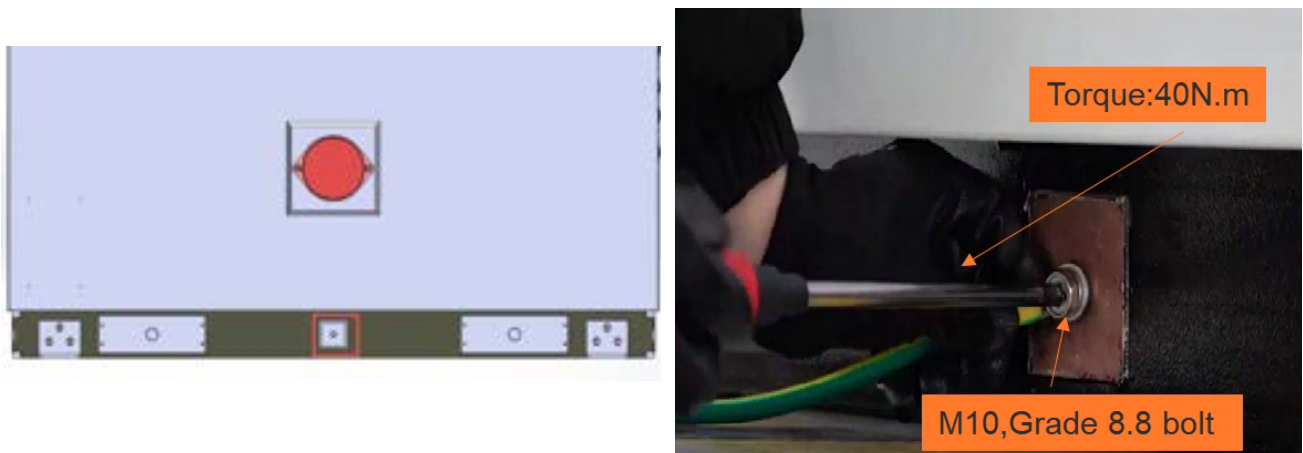
Figure 7-4 Cabinet ground connection
